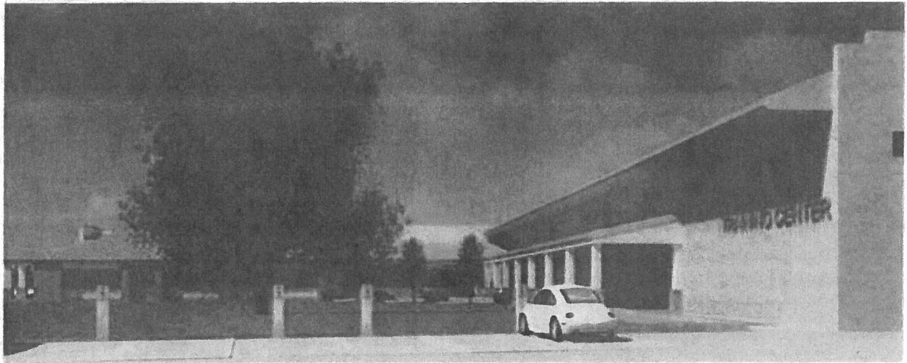
Student Parking (Southwest View)
