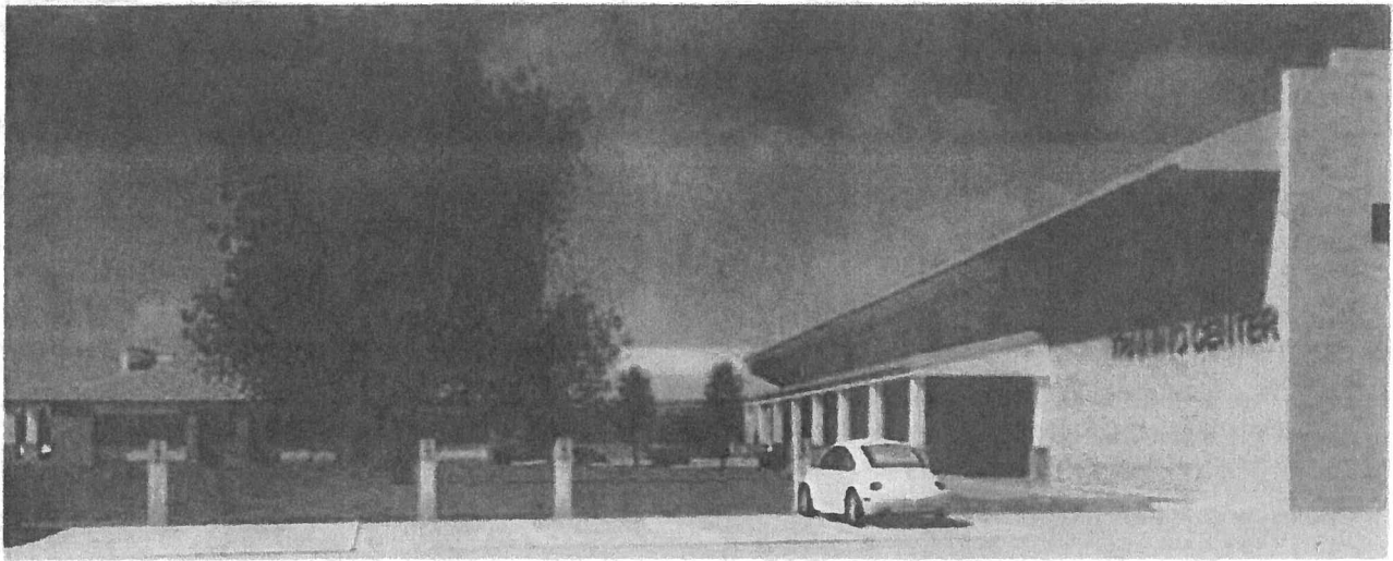
Student Parking (Southwest View)
